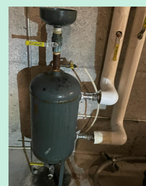
Figure 1: Pot feeder for a closed-loop chemical feed.
