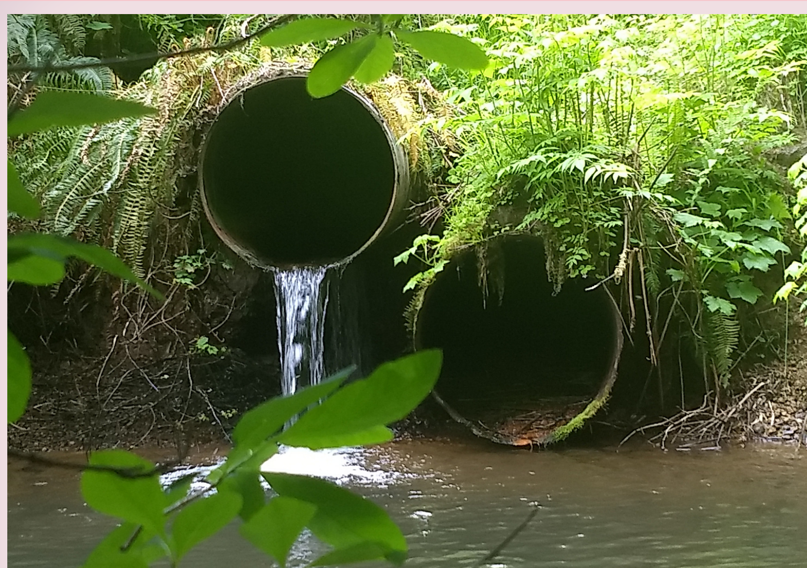
Figure 1: This picture shows how barriers prevent fish from traveling upstream.
