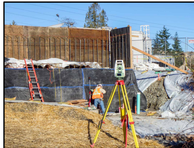
Fig 2: Below the tripod on the right of the photo there is a wooden marking stake and some biodegradable ribbons tied onto it. There is also blue eco-friendly survey paint showed in the image on the black wall.
